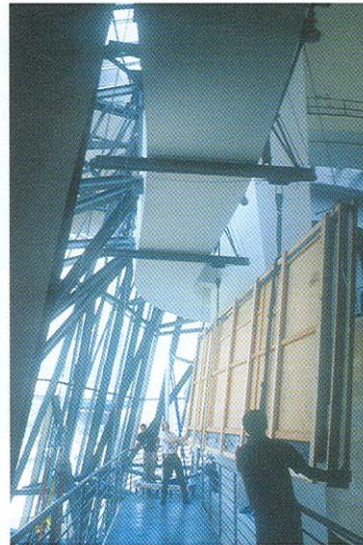
PLATE 7 A rig on the third-floor catwalk was used to lift Anselm Kiefer's Zweistromland to the second floor (p. 22).
